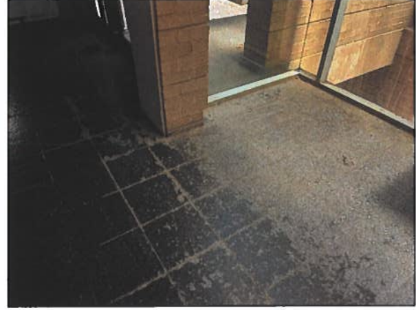
Figure 15: Sunlight damage on floor tiles in the Meyer Pienaar section of the Johannesburg Art Gallery.
