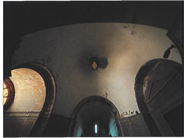
Figure 7: Continuous water ingress, visible over a large area in the movement spaces between exhibition halls.
