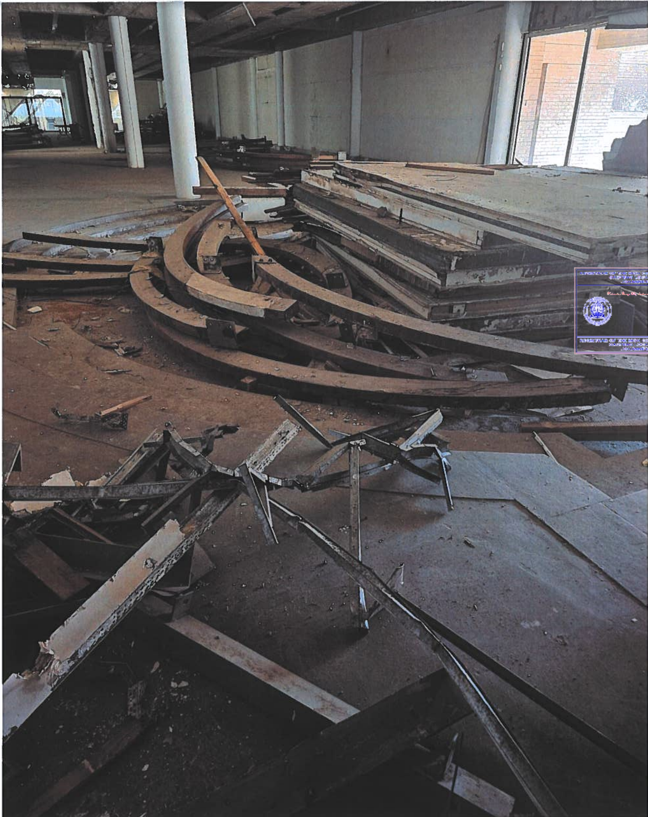
The award-winning Meyer-Pienaar gallery extension was 'renovated' under the watch of the Johannesburg Property Company in 2021. Copper roofs and vaulted ceilings were removed, and a concrete slab was thrown over the space. Structural engineers later found structural damage to the building, and the project to restore it was never completed. The
