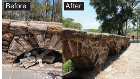
Stewart Drive Stonework stabilised and repaired
