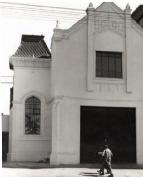
Presbyterian Church AKA Divine Bakery. 55 Mint Rd, Fordsburg. Architect G. Granger Fleming. Constructed 1897 as a church for Scottish residents, the space has retained its ecclesial architecture.
