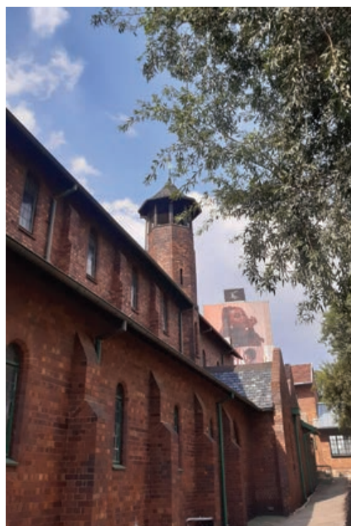
St Alban's Roof Restoration
