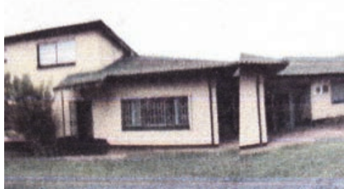
Chiefs House AKA Emakhosini. 7 Moroka Street, Meadowlands. Built in the late 1950s to accommodate homeland chiefs on their visits to urban areas.
