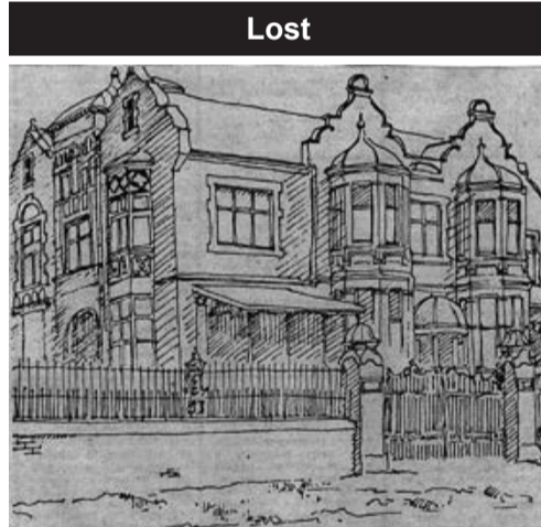
Barnato House AKA Dale Lace House / Norman Nursing Home. 103 - 111 Davies Steet, Doornfontein. Architect unknown. Constructed 1893. Demolished.
