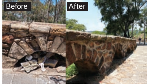
Stewart Drive Stonework stabilised and repaired
