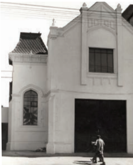
Presbyterian Church AKA Divine Bakery. 55 Mint Rd, Fordsburg. Architect G. Granger Fleming. Constructed 1897 as a church for Scottish residents, the space has retained its ecclesial architecture.
