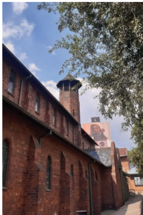
St Alban's Roof Restoration
