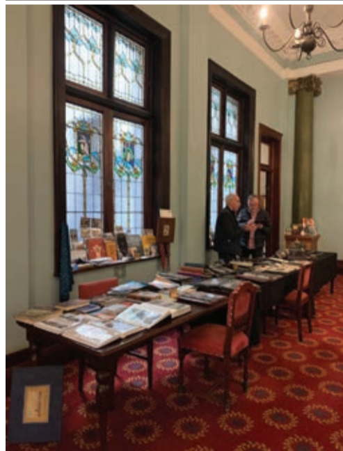
Rand Club , windows restoration
