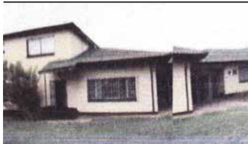
Chiefs House AKA Emakhosini. 7 Moroka Street, Meadowlands. Built in the late 1950s to accommodate homeland chiefs on their visits to urban areas.
