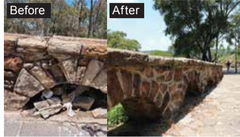
Stewart Drive Stonework stabilised and repaired
