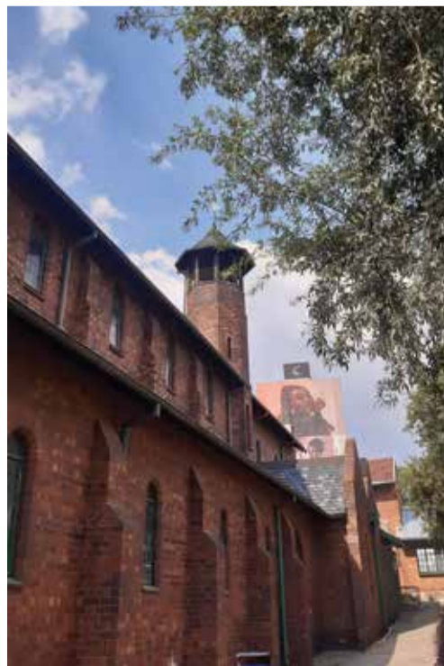
St Alban's Roof Restoration
